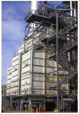
The design thermal efficiency of the heater was ~ 88% and was operating at 80- 81%. The stack temperature was almost  $300^{\circ}$ F higher than the design temperature.
