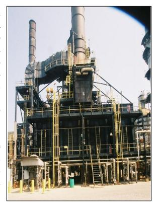
Furnace Improvements Services (FIS) performed an engineering study for NO<sub>x</sub> reduction on this furnace and modeled the furnace with Ultra Low NO<sub>x</sub> Burners. It was found that the radiant tubes in this heater had been suffering from high tube metal temperature and flame impingement. The convection section was inefficient and the air preheater operating temperature was reaching its metallurgical limits.
